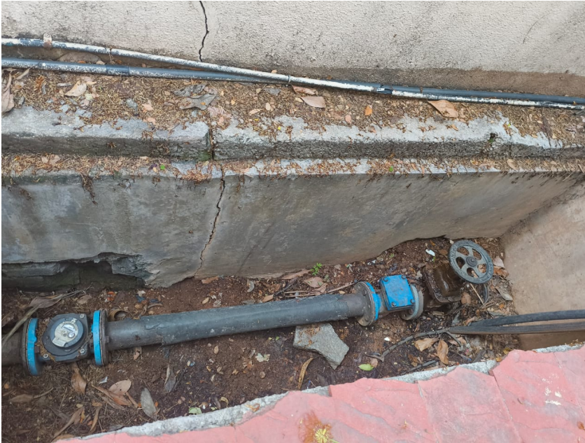
Fig 1 - The BWSSB water inlet valve, where water enters the apartment.
