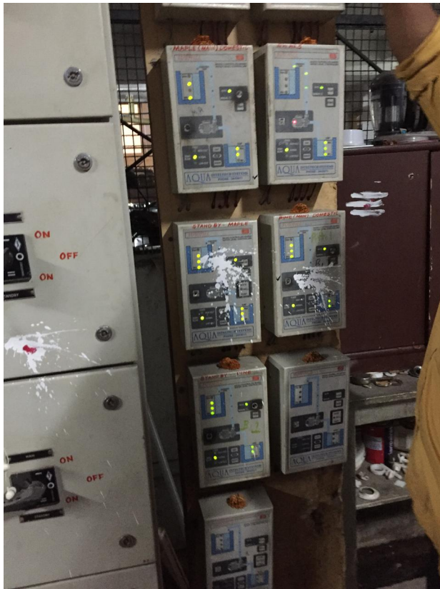
Fig 5 – Tanks are fitted with sensors that indicate water levels in them. Uncles operate the pumps based on these levels.
