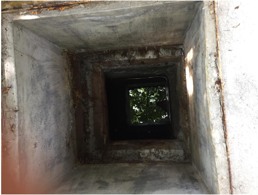
Fig 3 – The main domestic water sump – underground tank. It is below the play area. Most of us did not know that water is stored here. We wanted to go into the tank but Uncle did not let us. Water comes from the inlet valve into a fire tank and overflows into this. A fire tank is used in case of fire to pump water for firefighting.
