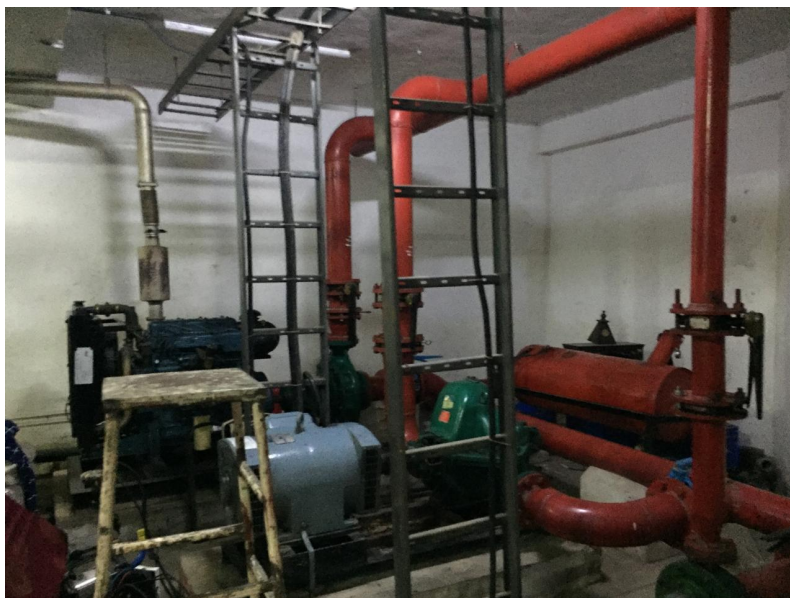
Fig 6 – Red pipes indicate fire safety. This pump operates the water from the fire tanks. A diesel generator and pump is kept ready since during a fire, power may be cut.
