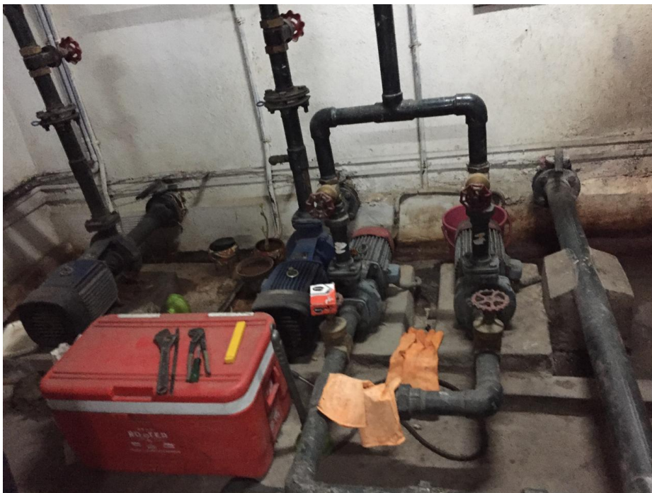
Fig 4 – The main pumps that carry water from underground sumps to overhead tanks. There are 4 such pumps that take water to four overhead tanks of the two blocks, Maple and Pine.
