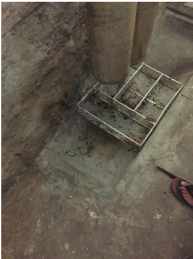
Fig 12 – Rainwater pipes from drains entering the basement area
