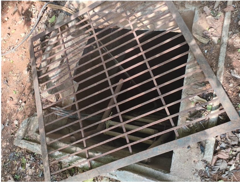
Fig 13 – Sewage tank. PGW used to have an old Sewage Treatment Plant. However that has not been functional for several years. The apartment has both grey and fresh water lines and separate tanks for each. However, this is not being used right now. Sewage water is being discharged into the BWSSB sewage lines.
